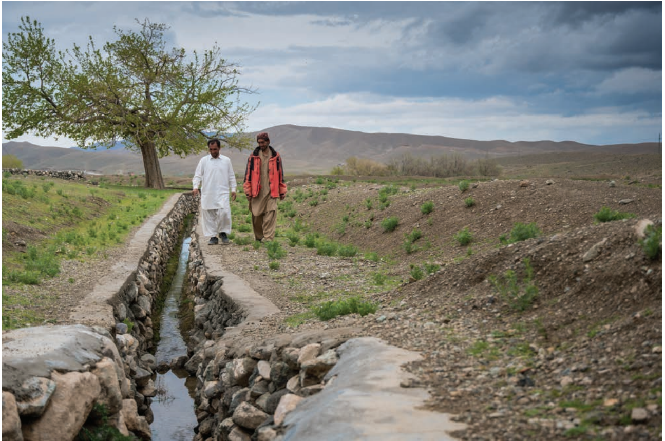
A karez cleaned and extended by Pak Village Organisation, in UC Khushab, Pishin
