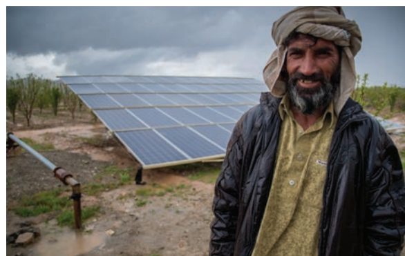
A solar water pump developed by a UC based organisation, Area Development Society, in UC Khushab, Pishin
