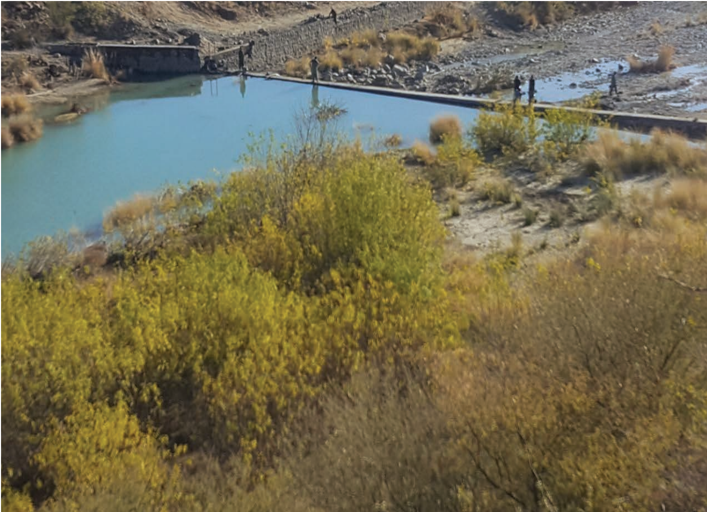
Weir construction for irrigation, UC Baiker, Dera Bugti
